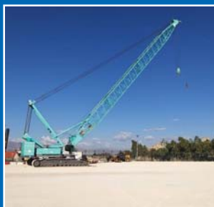
Crawler crane 250T
